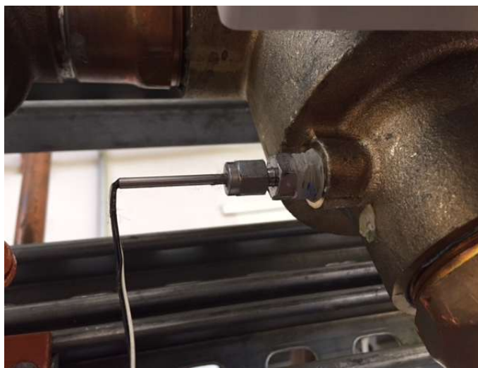
INSTALLATION OF COMPRESSION FITTING AND OUTLET RTD PROBE ON 2" PROTON VALVE BODY
